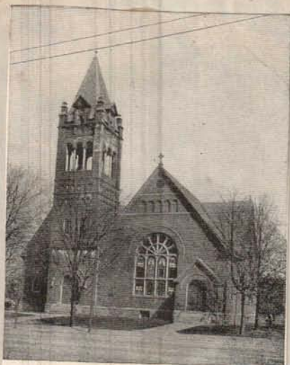
THE OLD CHURCH Dedicated 1891 Destroyed by fire January 6, 1925
