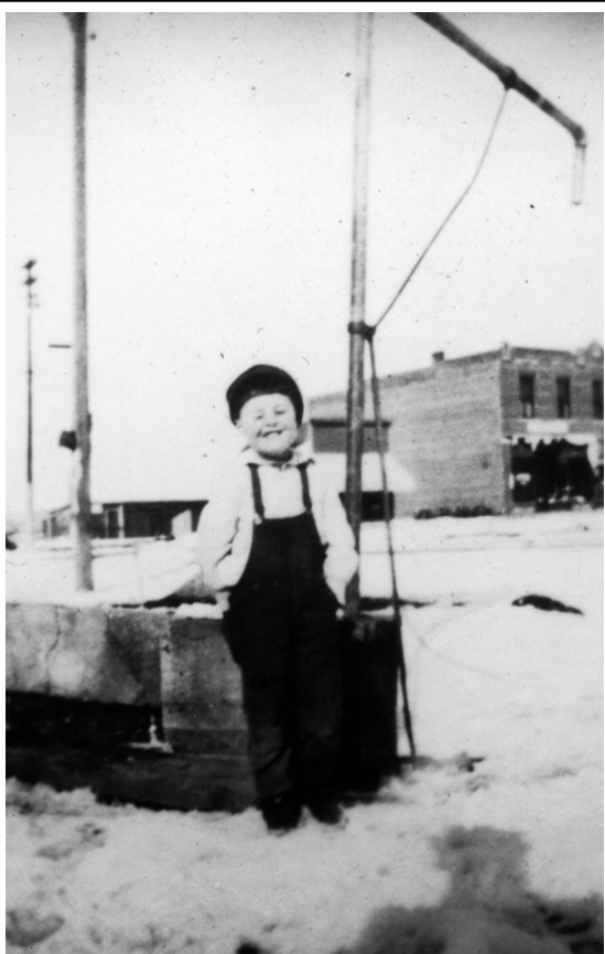
Water station at the corner of Harriett and Broad in July 1911, work started on the erection of a railroad water tank there.
