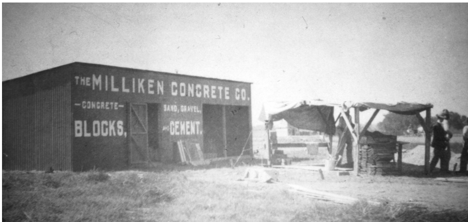
Milliken Concrete Company owned and operated by James B. Orman who was Governor of Colorado from 1901 - 1903. The blocks for the Cement Block Building were made there from sand and clay taken near the Thompson River.
