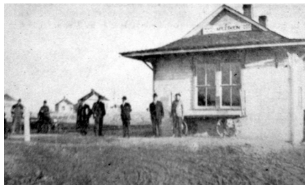
The Denver, Laramie & Northwestern Depot which was built in 1910. It was 24 ft x 60 ft., had two waiting rooms, a storage room and an office.
